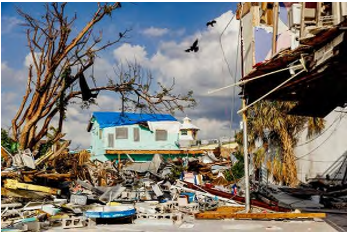
Demolished shops and restaurants in Fort Myers Beach, Fla. Credit...Scott McIntyre for The New York Times
