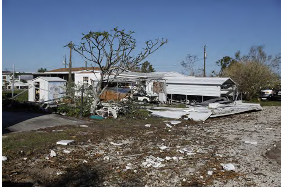
Debris from damage left by Hurricane Ian is seen in a mobile home park on Pine Island, Fla. on Oct. 28, 2022. Octavio Jones for NPR
