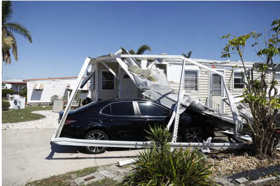
Debris from the damage left by Hurricane Ian is seen in a mobile home park in Fort Myers, Fla. on Oct. 27, 2022. Octavio Jones for NPR
