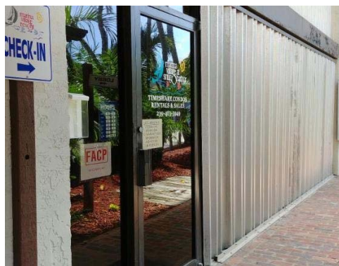
3 steps to installing the shutters
